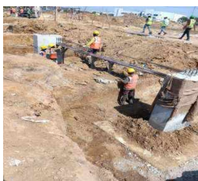
Plinth Beam Shuttering and Concrete Casting
