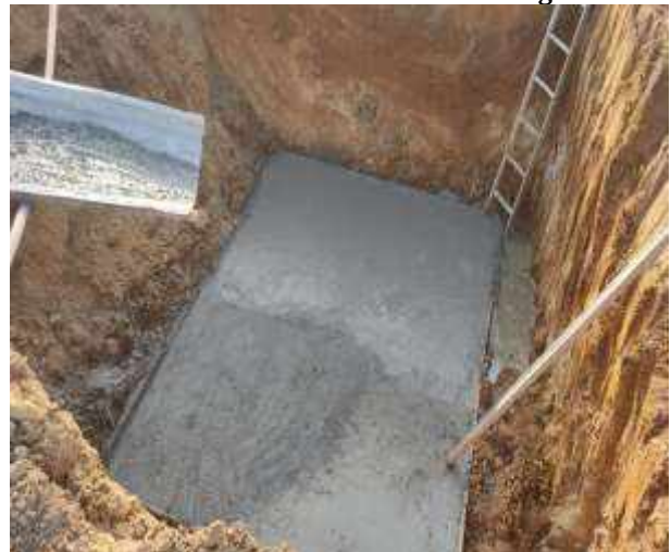
PCC Concrete Work
