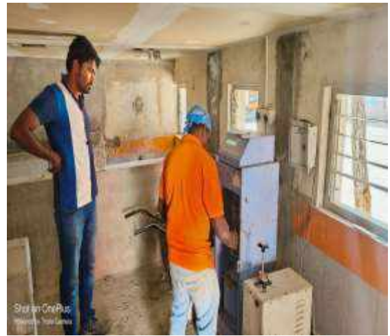
PCC Concrete Trial Mix Testing
