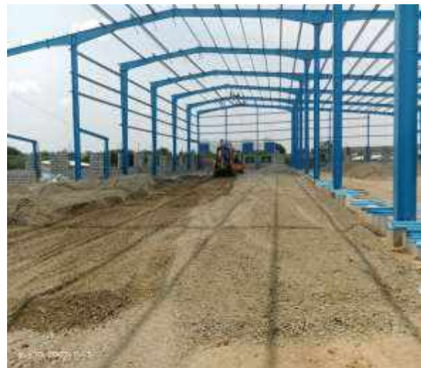
GSB Levelling and Compaction
