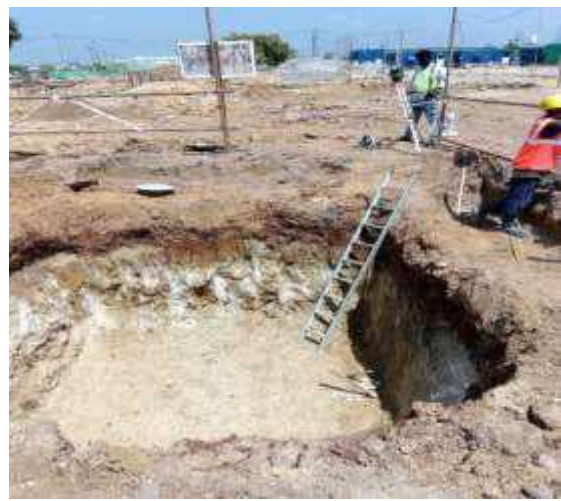
Footing Levelling and PCC Marking Work
