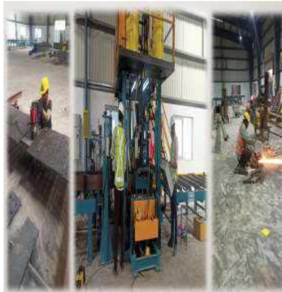
Civil Foundation Fabrication Work
