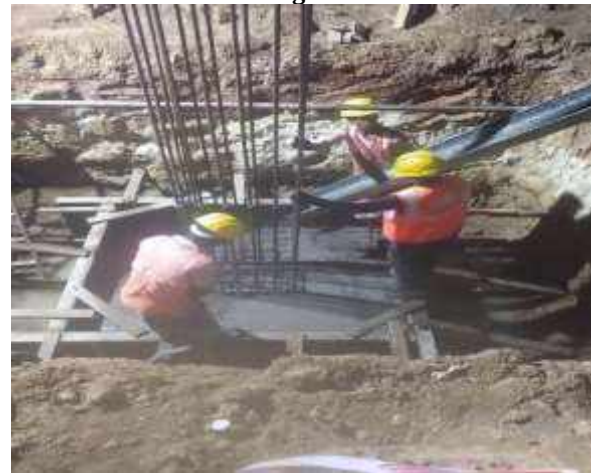
Footing Concrete Work, Pedestal Barbending & Shuttering
