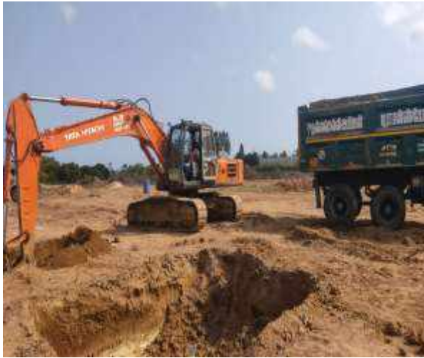
Earth work Excavation
