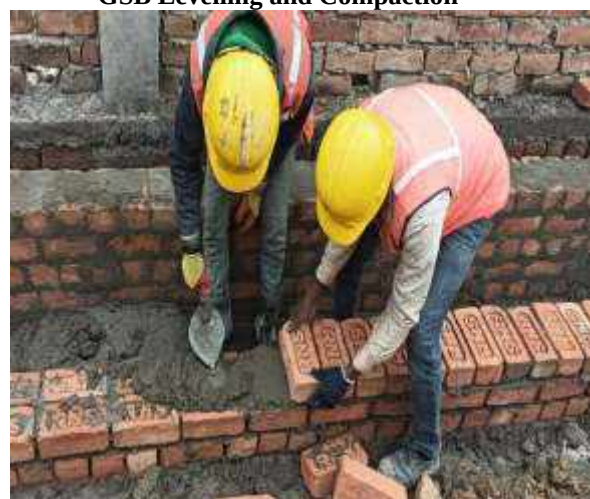
Brick/ Block Work
