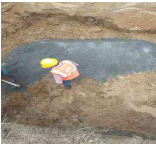
M- Sand Filling Work
