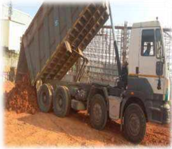
Soil Filling and Compaction
