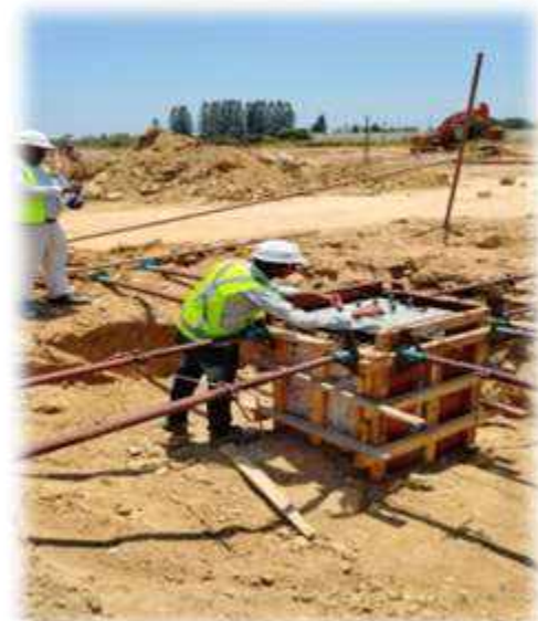
Anchor Bolt Fixing & Checking
