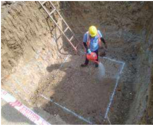
Anti Termite Work
